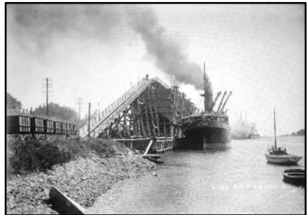
Lime Bins on the Devonport Wharf
